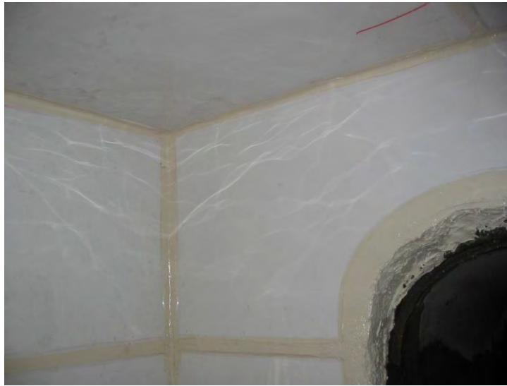
Figure 6-18. Junction Chamber Interior after Rehabilitation with the Two-Part System.
