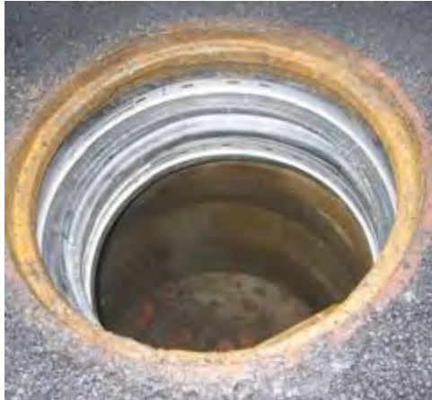
Figure 6-13. Example of a Rubber Internal Chimney Seal.
