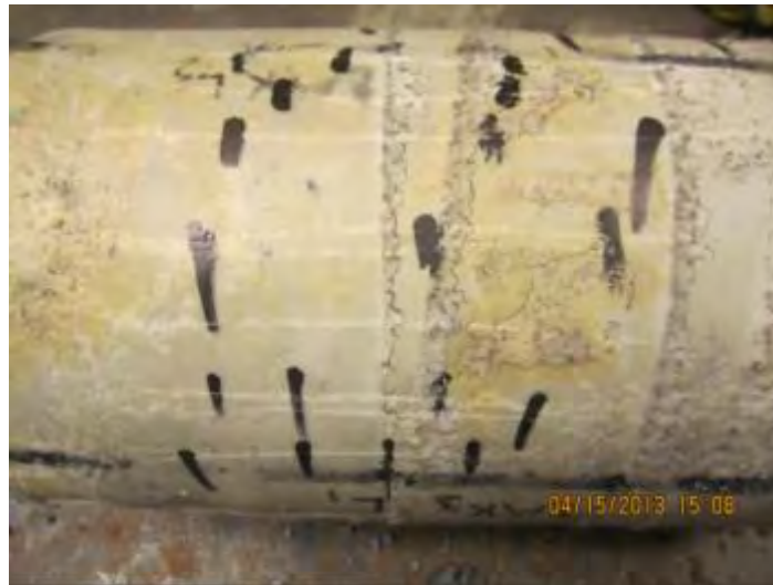
Figure C-36. Specimen CIP-C#3 at Failure, Note the Hairline Cracking.
