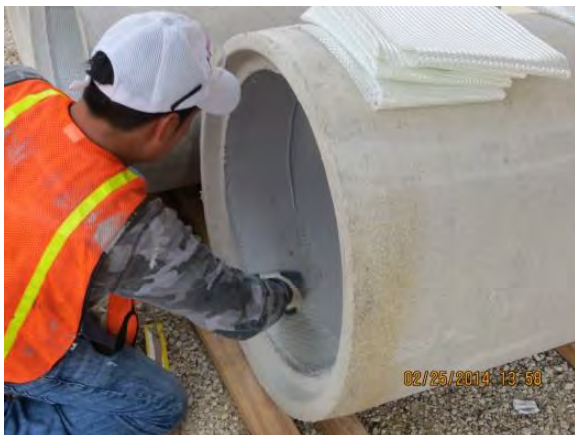
Figure D-1. Application of Epoxy over Glass Fiber.
