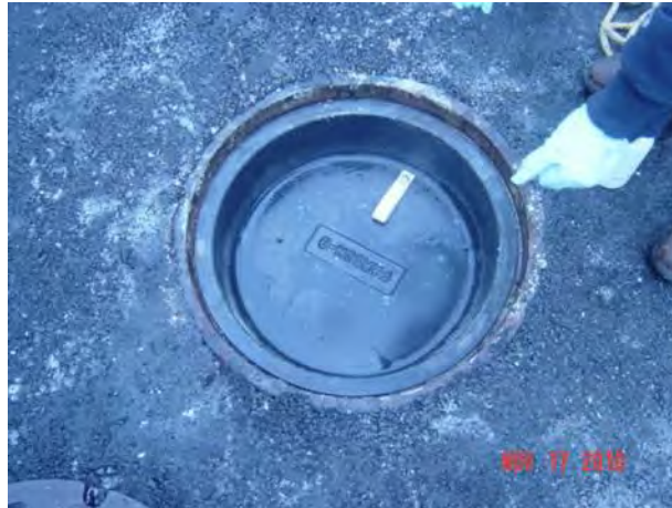
Figure 6-20. Inflow Dish (“Rain Stopper”) Inserted in a Manhole to Prevent Inflow Entering Through the Top Segment.
