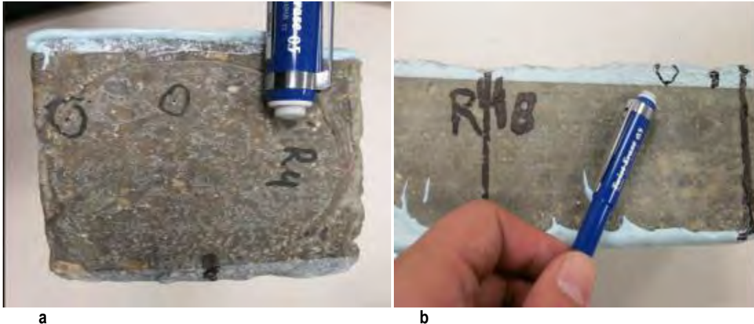
Figure C-6. Pinholes in the Concrete Substrate (a) and Liner (b).
