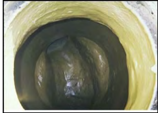
Figure 1-1. Manhole Rehabilitated with Cementitious Lining. Figure 1-2. Manhole Rehabilitated with Polymeric Lining.
