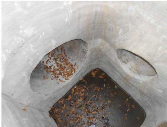
Figure 6-24. Manhole Lined with Calcium Aluminate Cement Liner.
