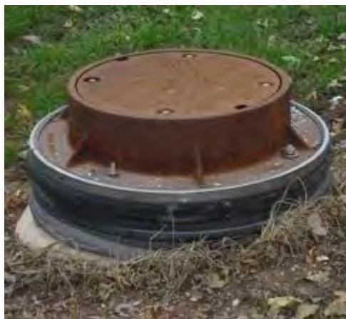
Figure 2-10. “Mechanical” Rubber Seal Applied Externally Source: Crete Specialty Products.
