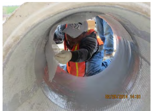
Figure D-2. Lining Using Glass Fiber.
