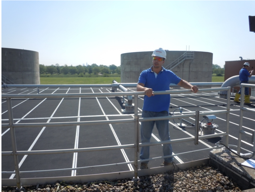
Figure 3. SNDR fixed Roof, jet pump discharge and air supply line
