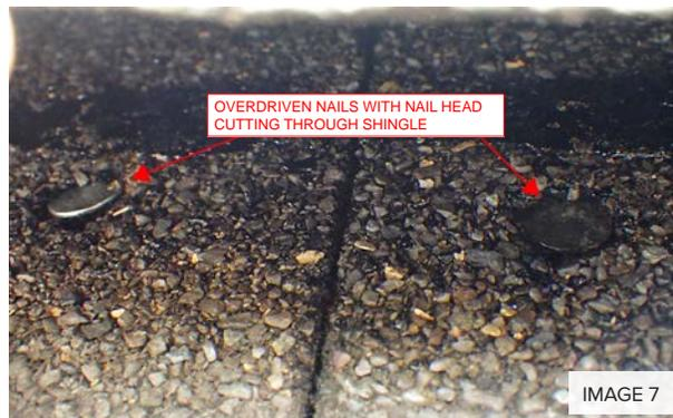
The previous list of questions is not an all-inclusive list of things to be on the lookout for, but it is a good starting point when shingle slippage is a possibility. Though we have focused on laminated asphalt shingles, similar slippage conditions can also exist on tabbed shingles, such as the common three-tab shingle.
