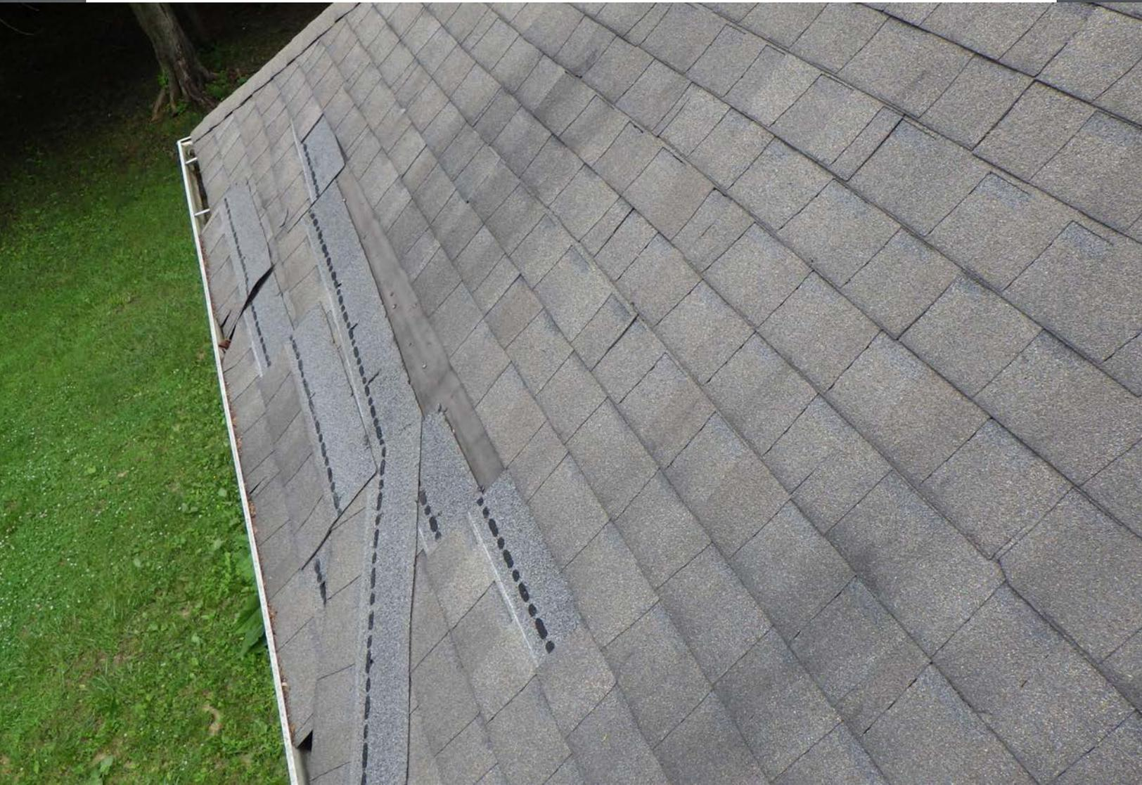
Have you ever inspected a shingled roof and wondered why the shingles have slipped out of place? Was it the result of wind forces, or could the placement of the nail or staple fasteners have had anything to do with it?
