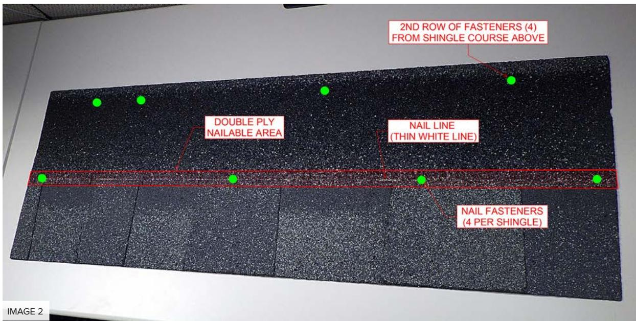
Standard shingle installation includes four fasteners per shingle within the nailable area, with fasteners approximately one inch from each end and the remaining two fasteners near the one-third points (Image 2). With the shingles installed in an overlapping fashion, each shingle will end up with a second row of fasteners attaching them to the roof deck and, therefore, eight total fasteners per shingle (Image 2).
