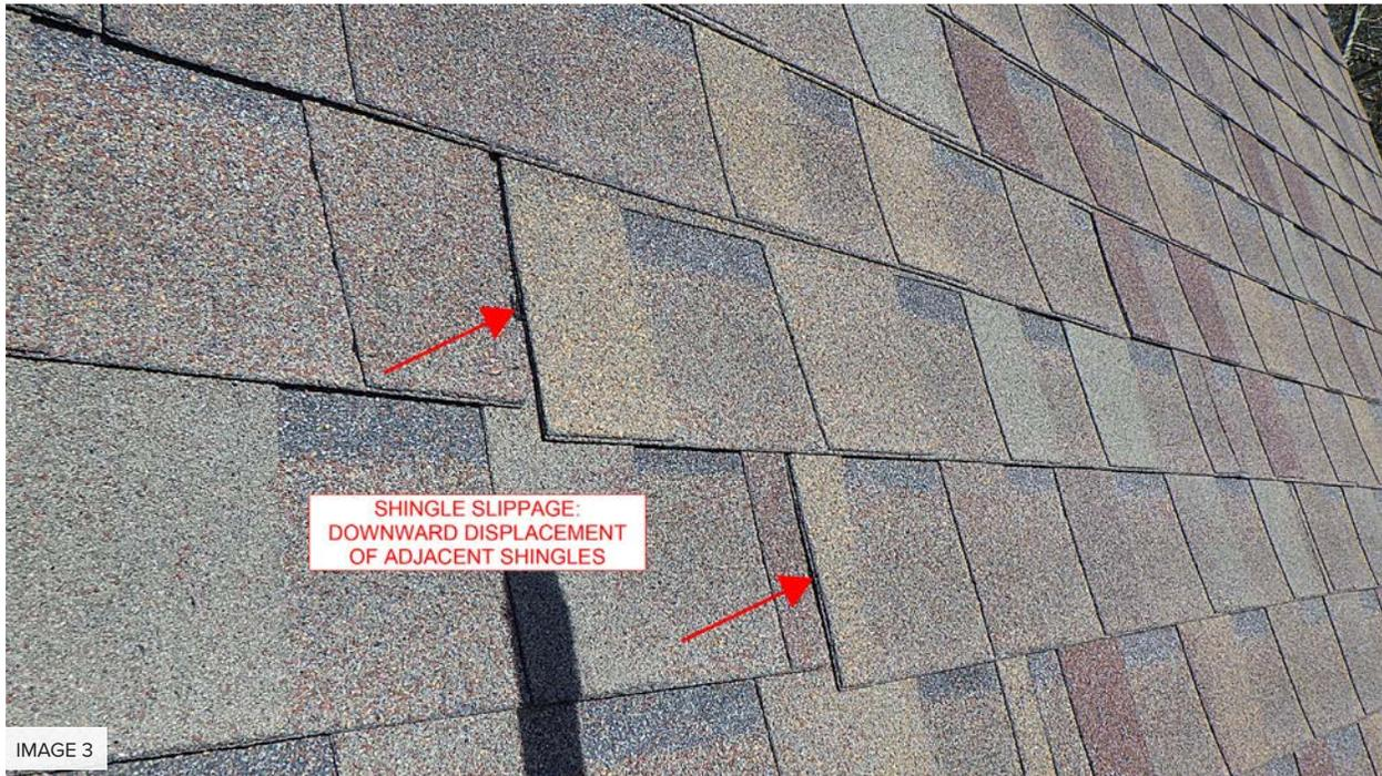
Now that we've reviewed some of the basics of laminated shingles and how they are attached to the roof deck, let's consider an issue we commonly observe on wind assessments (and commonly see misidentified as wind damage)—slipped shingles (see Image 3). Slipped shingles are those shingles displaced from their original position on the roof due to fasteners being improperly located and/or overdriven and thereby having a reduced or nonexistent attachment to the roof deck.
