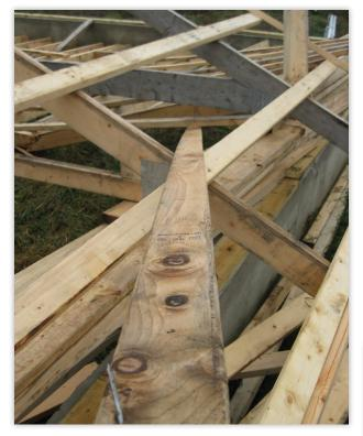
The rectangular barn was approximately 40 feet by 80 feet (long dimension in the east-west direction) and was constructed of common wood framing with wood roof trusses supported by wood stud walls that stood on short concrete foundation walls. The woodframed barn was situated in an open field and was approximately 70 percent complete at the time of the collapse, lacking wall siding and approximately 25 percent of the metal roofing.
