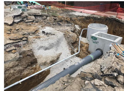
Storm Sir 11 and 11A and 2" PVC Conduit Installed for G.I. Control Valve
