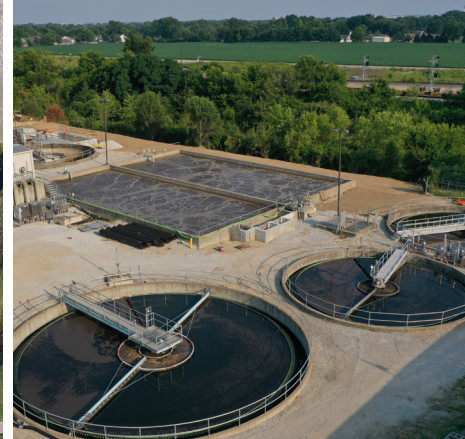
Hendricks County Regional Sewer District Wastewater Treatment Plant Expansion Progress Design-Build, Avon, Indiana
