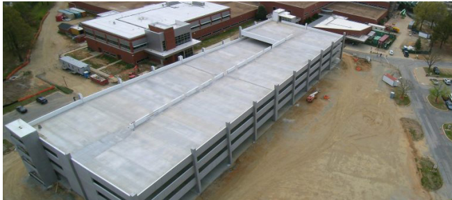
HH McGuire VA Medical Center Parking Garage, Richmond, Virginia
