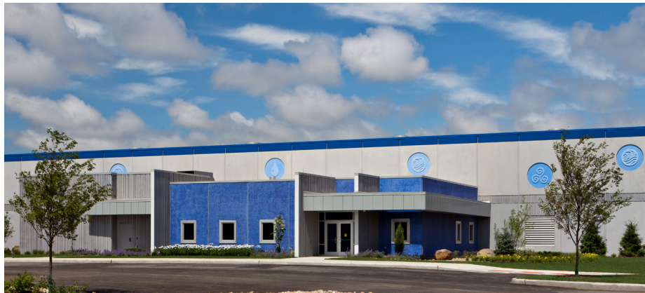
Water Treatment Plant, East Chicago, Indiana
