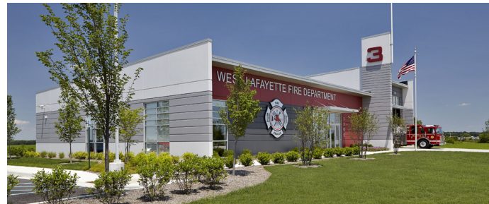
Fire Station No. 3 Purdue Research Park, West Lafayette, Indiana
