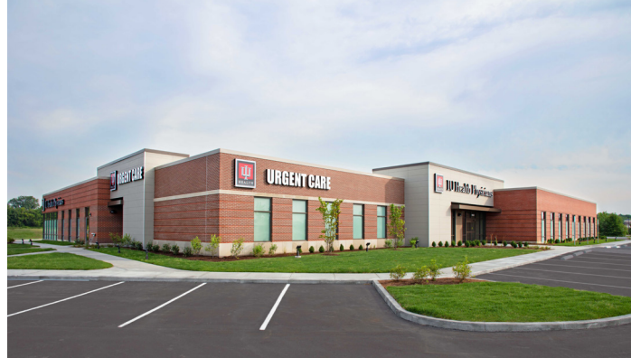
Indiana University Health Medical Office Building, Noblesville, Indiana
