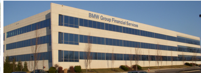
BMW Group Financial Services Building, Hilliard, Ohio
