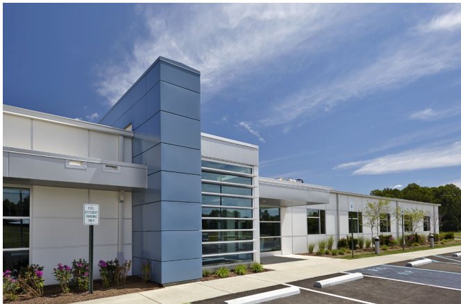
Battery Innovation Center (BIC), Crane, Indiana
