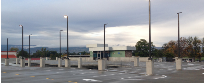
Western Colorado VA Medical Center Parking Structure, Grand Junction, Colorado
