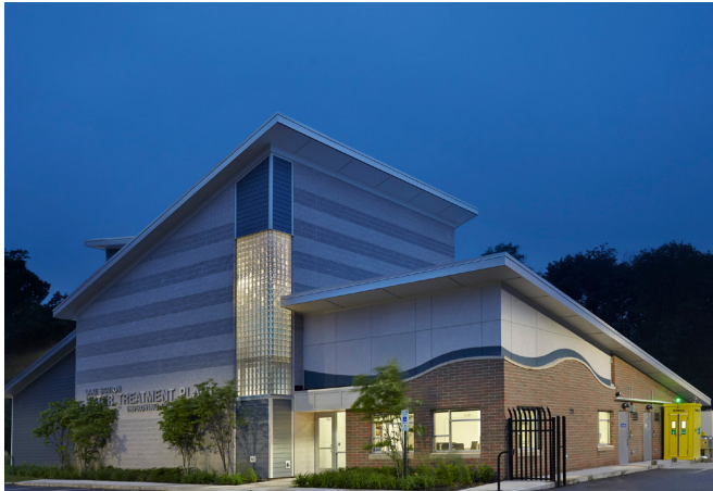
Water Treatment Plant, Lake Station, Indiana
