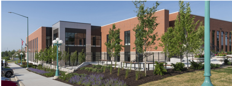
Noble County Annex Building, Albion, Indiana
