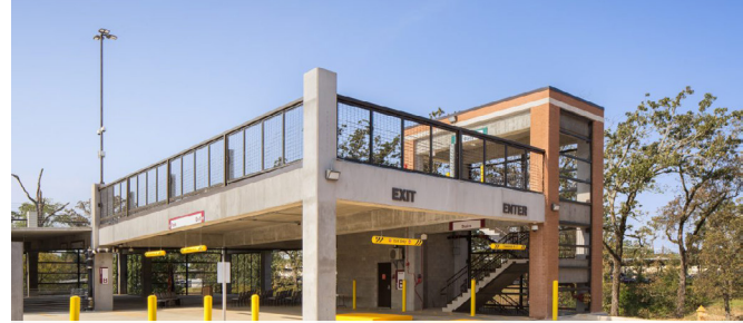
Overton Brooks VA Medical Center Parking Structure, Shreveport, Louisiana
