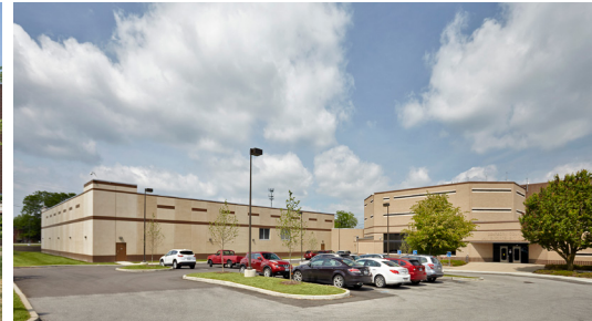
Dearborn County Jail Renovation, Lawrenceburg, Indiana
