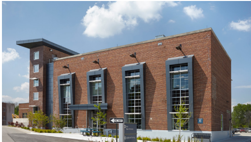
Lutz VAMC Building 6 Adaptive Reuse, Boilerhouse to Office Conversion, Saginaw, Michigan
