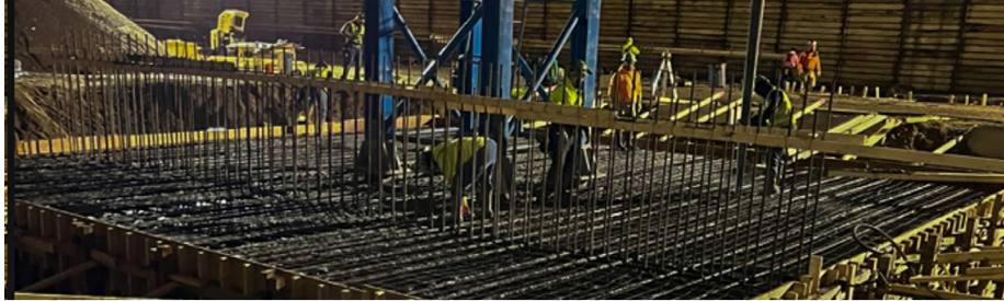
Messer Construction Tower Crane Foundation, Indianapolis, Indiana
