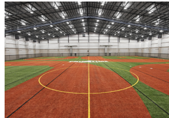
Finch Creek Park New Fieldhouse, Noblesville, Indiana
