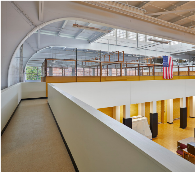
Purdue University Lambert Hall Platform Renovation, West Lafayette, Indiana
