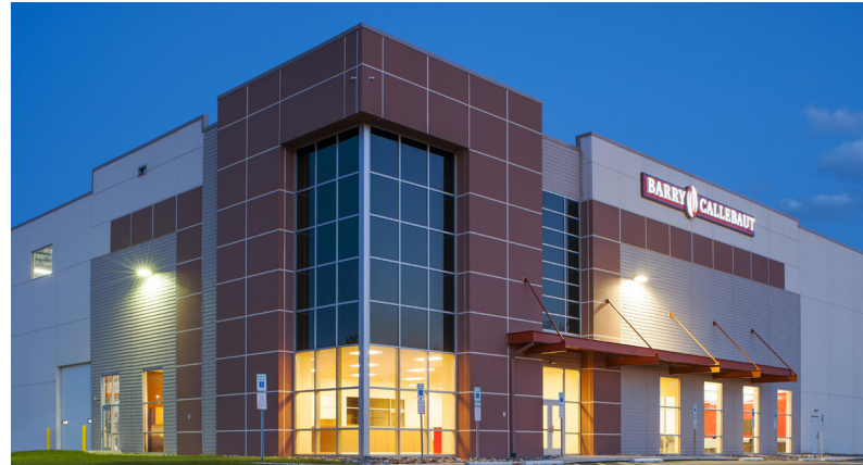
Lehigh Valley Trade Center Lower, Nazareth and Bethlehem Township, Pennsylvania
