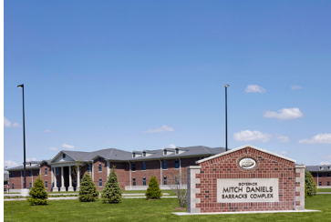
Indiana National Guard Mitch Daniels Barracks Complex, Camp Atterbury, Indiana
