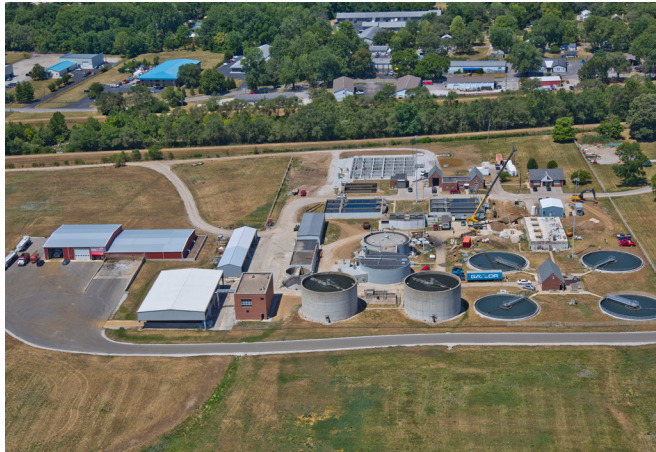
UNOX and Biosolids Upgrade, Speedway, Indiana
