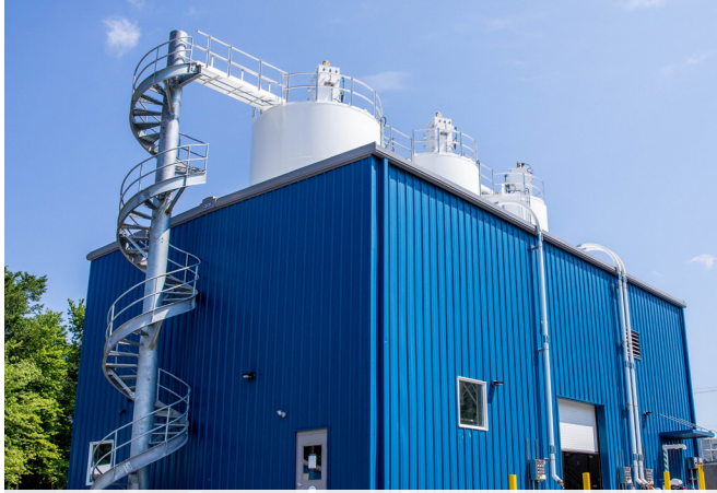
Struthers Water Treatment Plant, Poland, Ohio
