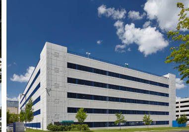
Veterans Affairs Parking Structure and Vertical Expansion, Indianapolis, Indiana
