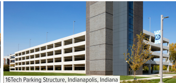
16Tech Parking Structure, Indianapolis, Indiana
