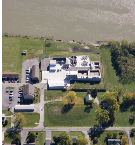
Wastewater Treatment Plant, Rising Sun, Indiana
