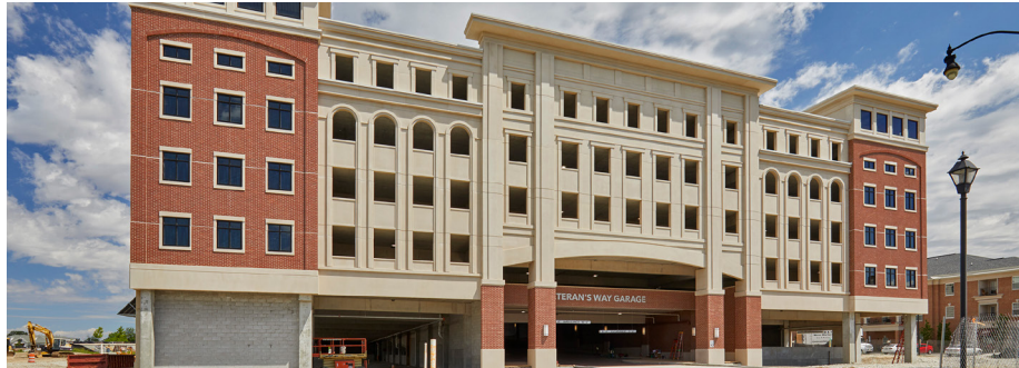
Carmel Park East Parking Structure, Carmel, Indiana
