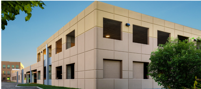
Garrison Parking Garage, Carmel, Indiana
