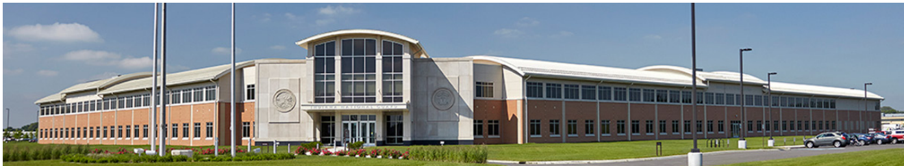
Stout Field National Guard Joint Forces Headquarters Addition, Indianapolis, Indiana
