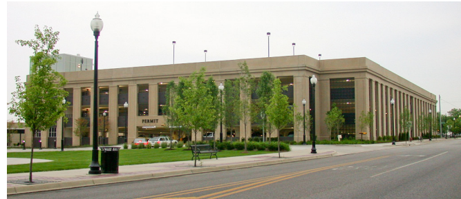
Cooper and Francs Parking Decks, Jackson, Michigan
