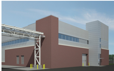
Allison Transmission Boiler Building, Indianapolis, Indiana
