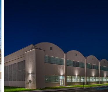
Wright Patterson AFB Hangar 6 Office Conversion, Dayton, Ohio
