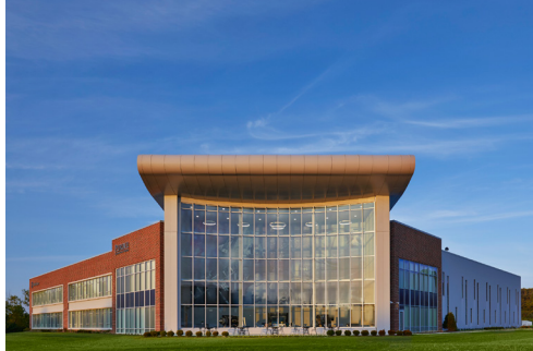
Purdue Research Foundation Aerotech Flagship Building, West Lafayette, Indiana
